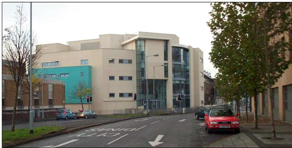
The Llewelyn Tower Block – Viewed from Alexandra road
